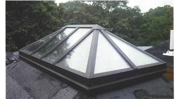
Materials count. A skylight or sunroom must withstand wind, rain and sun, so even a simple project demands a dimensionally stable frame. The best domestic woods are clear, vertical-grain redwood and cedar (photo below). Outside, hips, valleys and angles can be covered with custom aluminum caps that can be fabricated at a sheetmetal shop (photo right). They're held in place by exposed stainless-steel screws with gasketed washers.
